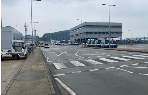
B T5 Southern Service Road
