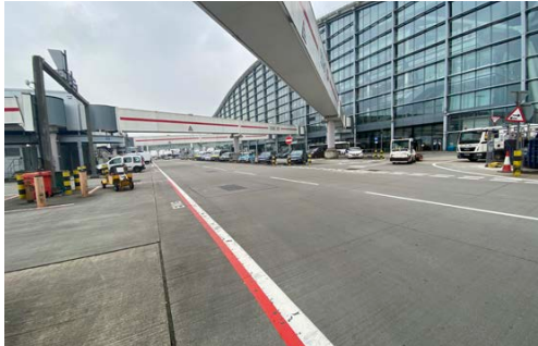
A T5 Terminal Approach Road North
