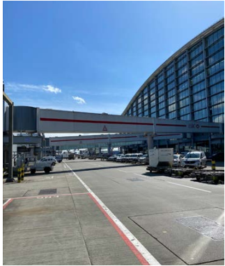
A T5 Terminal Approach Road North
