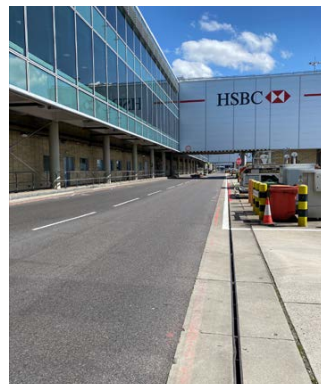
C T3 Pier 6 Road South
