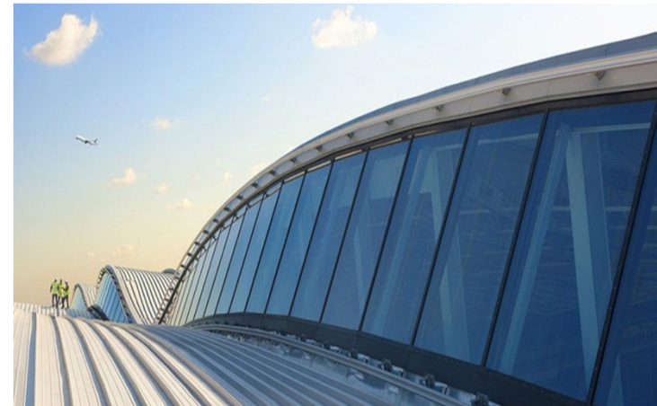
Roof of main Terminal 2 building
