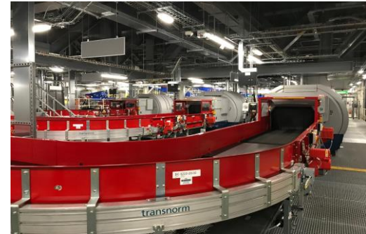
T5 HBS replacement
