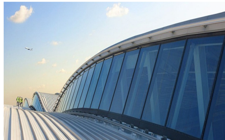
Roof of main Terminal 2 building
