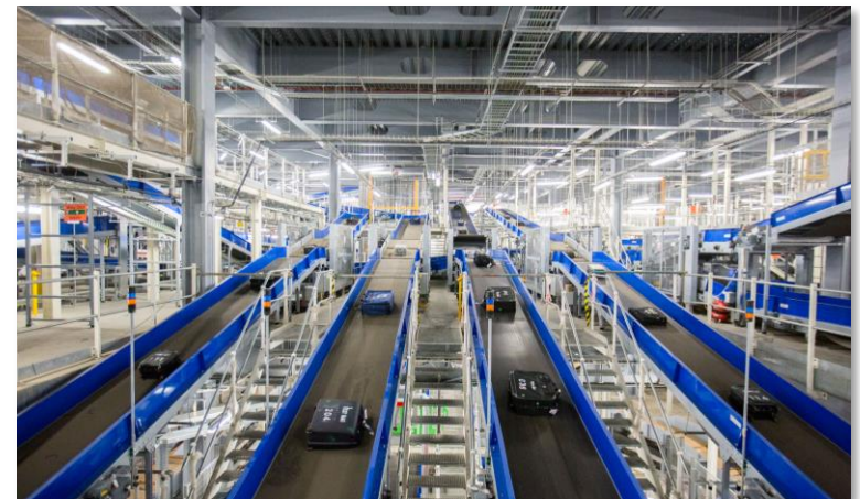
Terminal 3 Integrated Baggage facility
