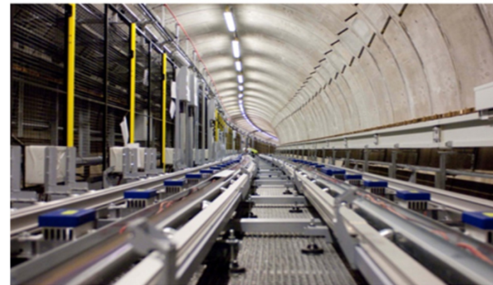
Terminal 3-5 baggage tunnel
