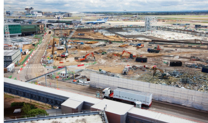
Terminal 2 site – August 2010
