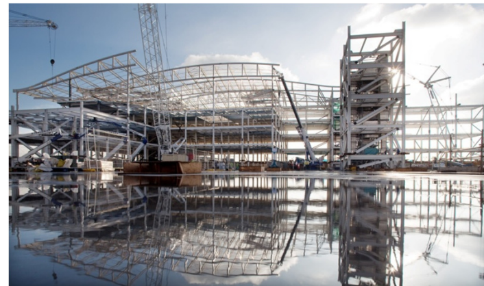
Terminal 2 site – January 2011
